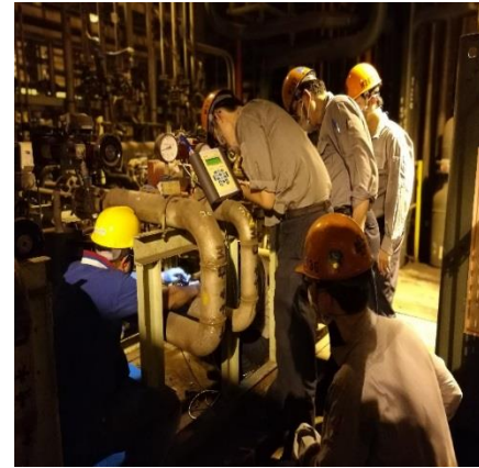
連鑄冷卻水 3" CS pipe (w/ scale \text{CaF}_2 )
