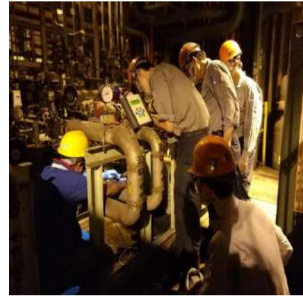
連鑄冷卻水 3" CS pipe (w/ scale \text{CaF}_2 )
